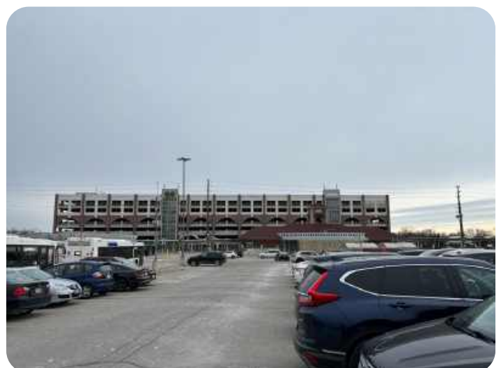
Oakville GO Bus parking structure
